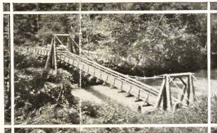
Thunder Creek suspension bridge
